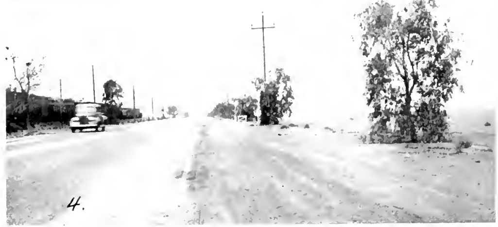
1—Looking North along center line of proposed new 4-lane divided highway North of Bakersfield. 2—Present State highway will become southbound roadways of new highway. 3—Existing trees will form a screen between the two roadways. 4—Trees on right have been permitted to grow down to ground to form screen.
